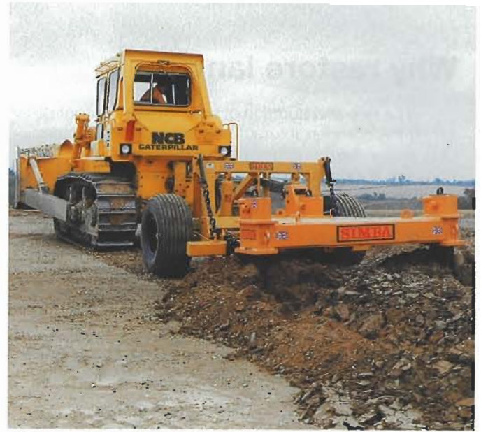
Fig. 30. Breaking up the surface of the infill material (prior to restoration of subsoil and topsoil) to improve drainage.
