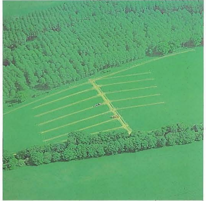
Fig. 22. 'Herringbone' pattern of a newly laid drainage system, as seen from the air.
