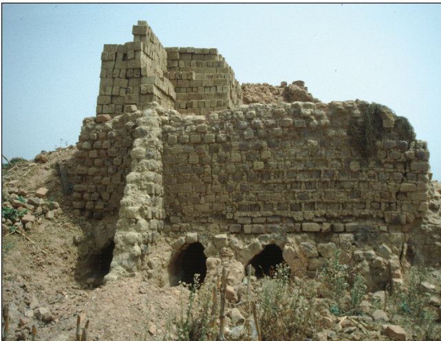
Mud bricks used for construction in Mali (AB).
